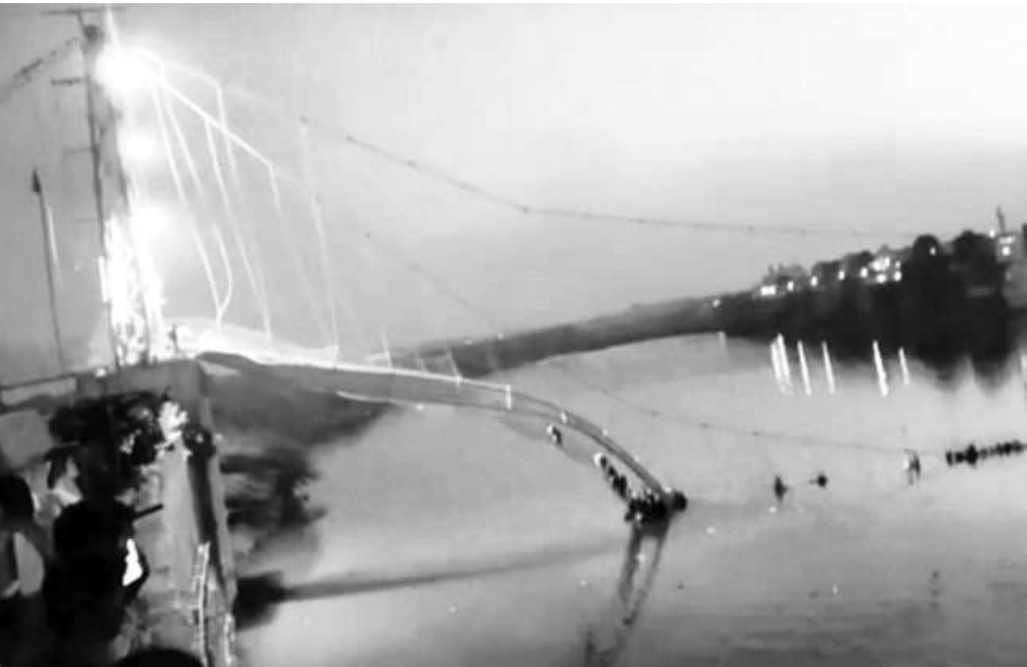
The collapsed portion of an old suspension bridge over the Machchhu river, in Gujarat's Morbi on Sunday
